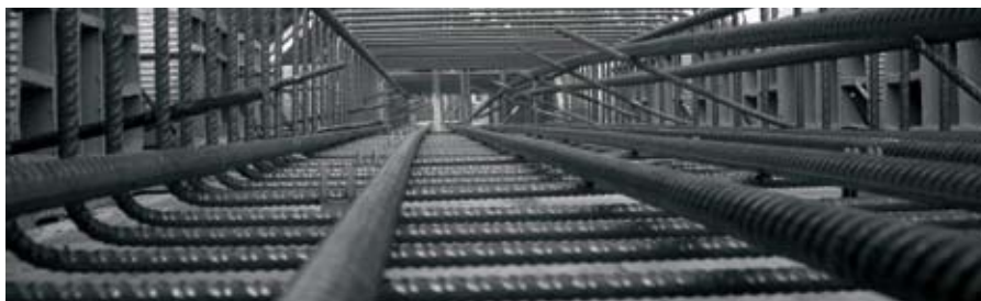
Joint reinforcement • Armature du noeuds
