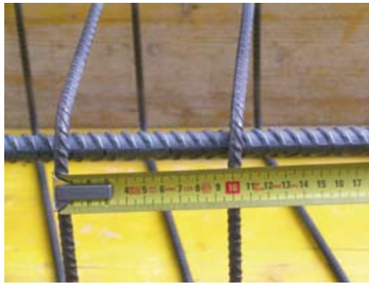
Joint reinforcement • Armature du noeuds
