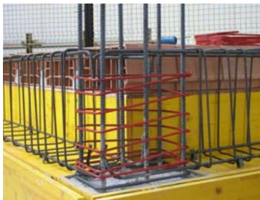
Joint reinforcement • Armature du noeuds
