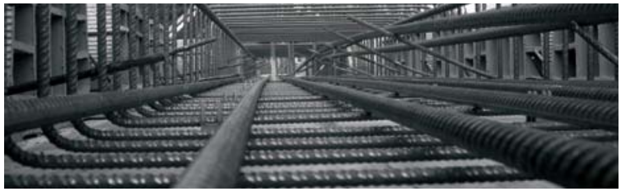
Joint reinforcement • Armature du noeuds
